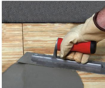
**Ash Grove Pro® Skim Patch is a trowelable Portland cement based patching compound for use as a quick-setting floor underlayment.**
