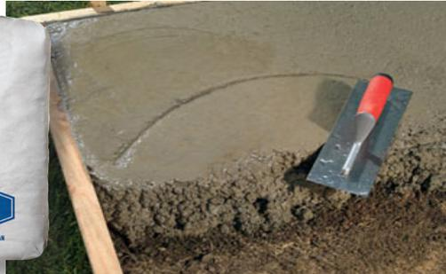
**Ash Grove® Crack-Resistant Mix is a uniformly blended mixture of portland cement, sand, rock, reinforcing fibers and other special additives specifically engineered to provide superior resistance to cracking and shrinking.**
